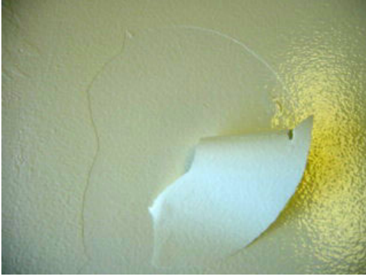
FIGURE 3, Poor Intercoat Adhesion.
